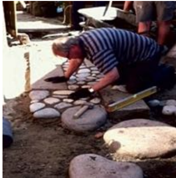
Building the nobedan path
