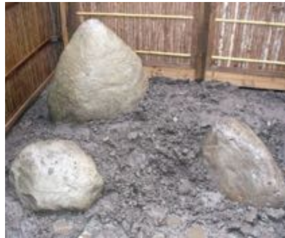
Entrance to garden - under construction
