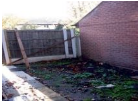
Site for garden - Front entrance
