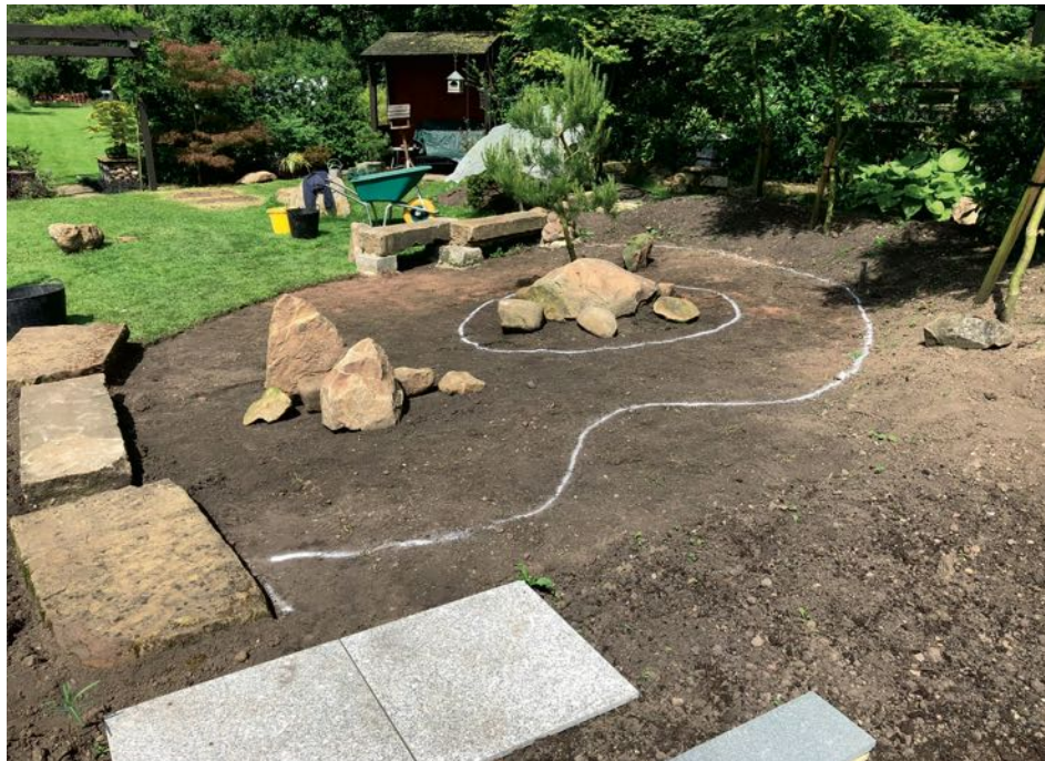
Figure 1: Area for gravel with turf removed and temporary placement of stones.
