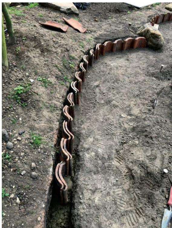
Figure 3: Edging of double clay pantiles in progress.
