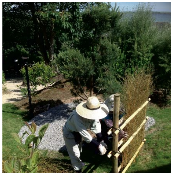
Figure 8: The tea garden in the 'Arrival in Japan' section was designed and constructed by Kyoto master gardener, Kazuki Kusumi. Here he is constructing Chasen-gaki ("tea-whisk") fence.
