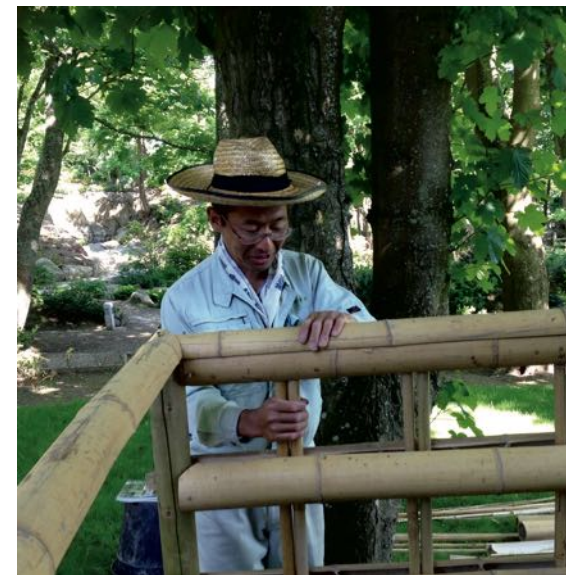
Figure 9: Here Kazuki Kusumi is constructing a yotsume-gaki fence.
