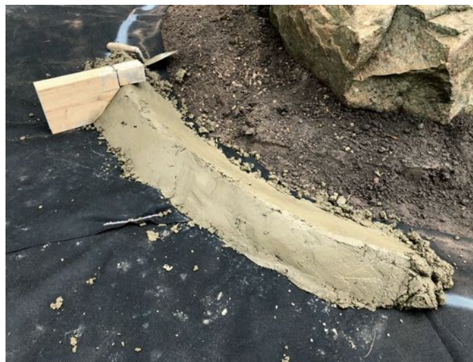
Figure 4: Mortar fillet with template.
