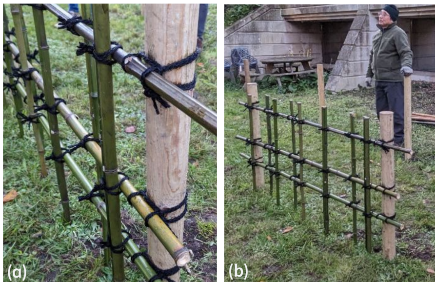
Figure 7: (a) Detailed view of the knots and (b) the completed six foot long yotsume-gaki section. Note: for this demonstration fence the do-bachi ends are not mitred and screwed into the bashira .
