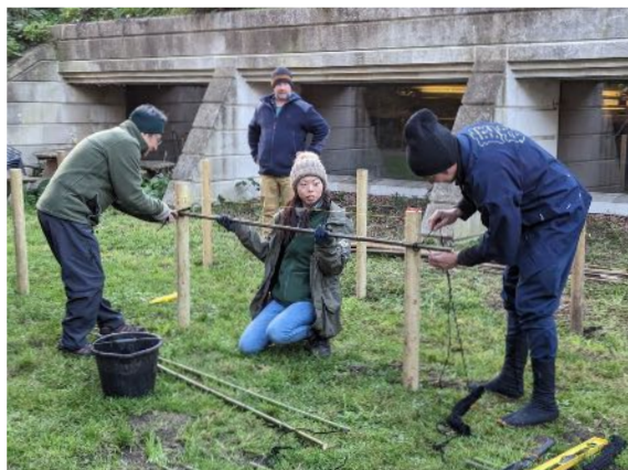
Figure 4: Checking the do-buchi (horizontal pole) is level before using twine to attach it to the oya-bashira (end posts).
