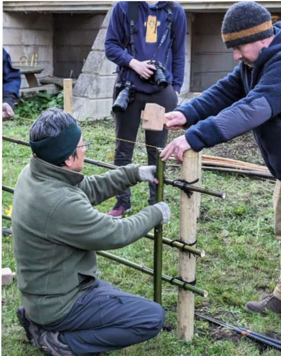
Figure 5: Knocking the tate-ko (vertical pole) into the ground until the top line lines up with the string before knot tying.
