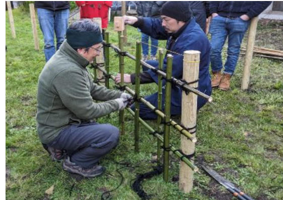
Figure 6: More tate-ko (vertical poles) are then attached on alternating sides of the do-buchi (horizontal poles).
