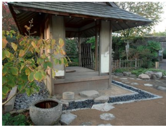
The new roof drainage channel November 2018.
