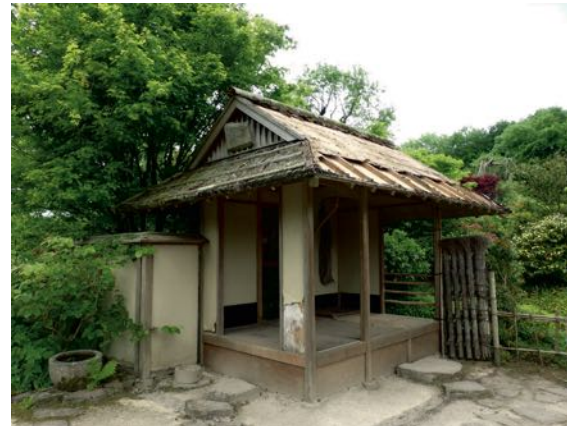
The tea-house in July 2016.
