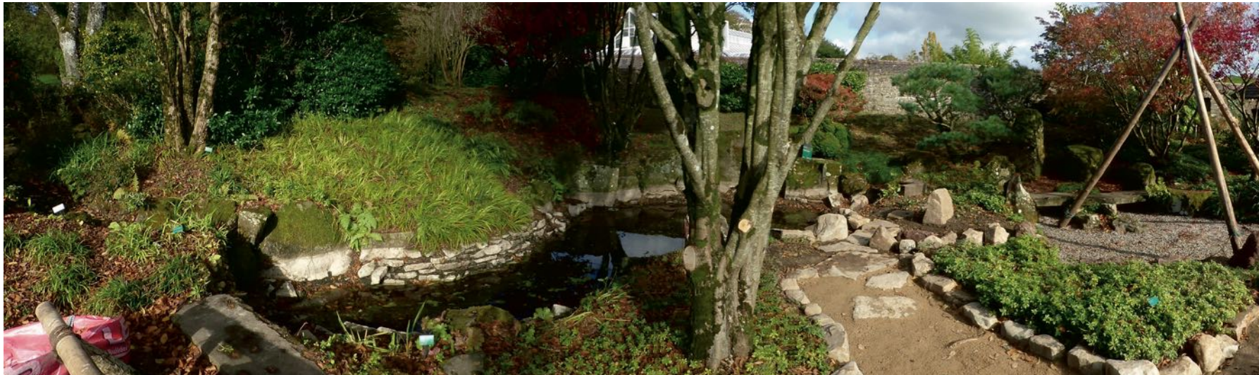
Work in progress October 2018.
